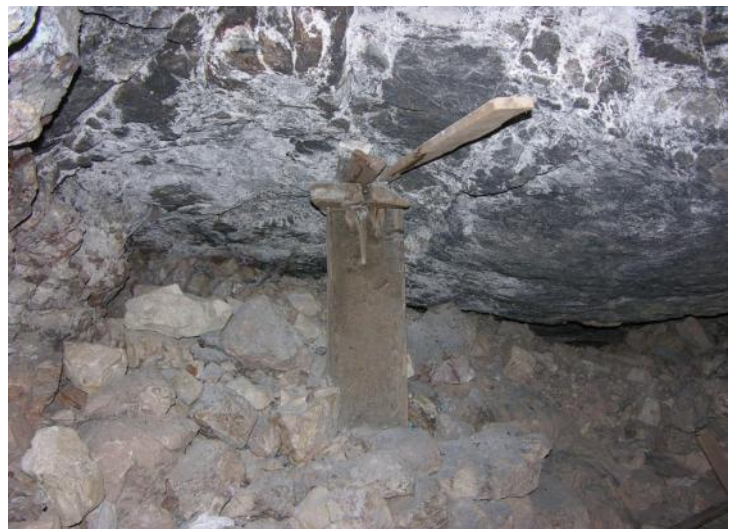
Timbering in the Arsenate Drift of the Silver Coin Mine
