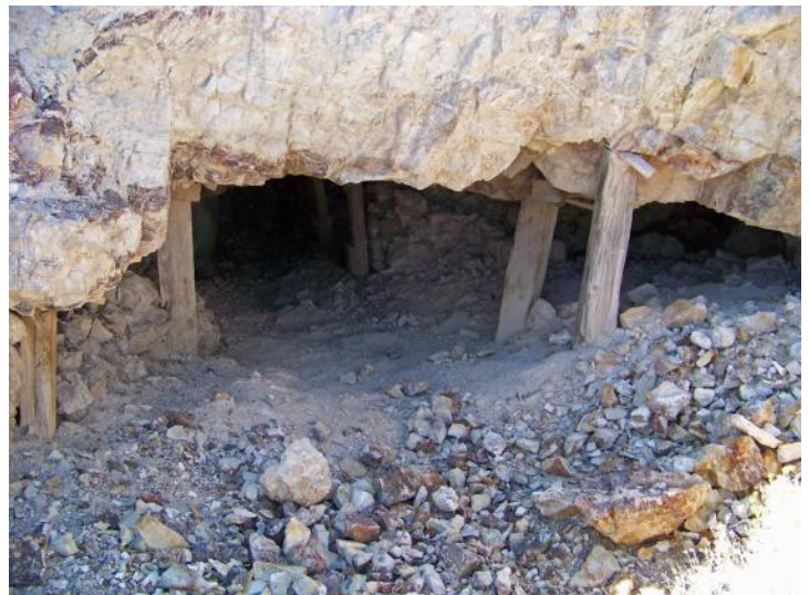
The Decline to the Arsenate Drift at the Silver Coin Mine—what is missing in this photograph is scale and slope. The decline tunnel is about 3 ½ to 4 feet tall, slopes at a moderately steep angle, and the floor is loose rubble—
