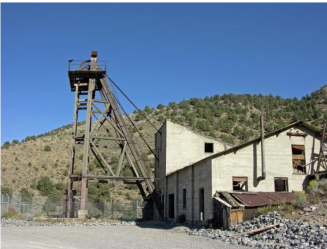
The Headframe and Hoist Building at the Eagle and Blue Bell Mine
